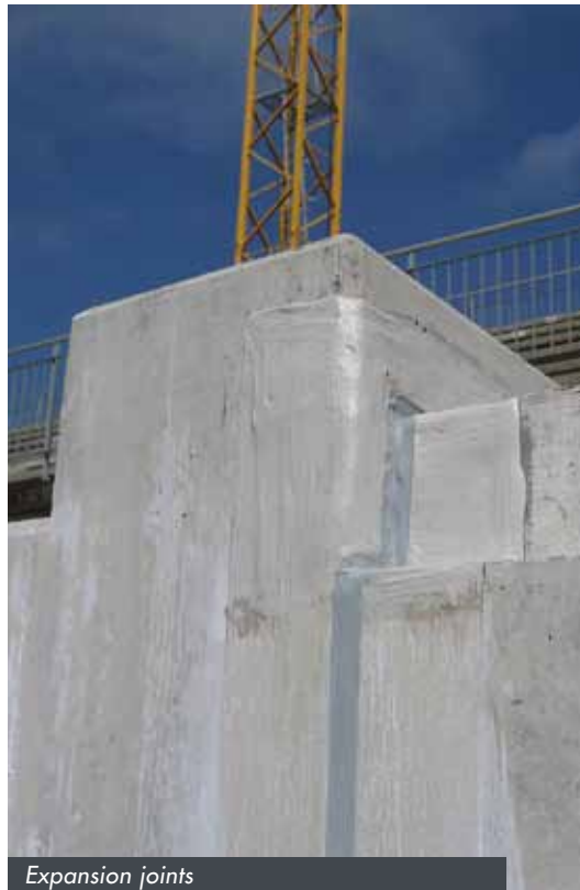
Construction joints
